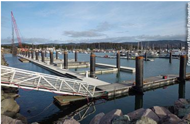
March 2014: Rebuild in "tsunami resistant" Crescent City Harbor
